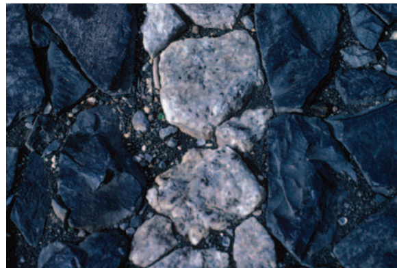
FIGURE 1. Carbonatite clasts make up the centre line of the road (top picture). Black paving stones are basaltic cobbles. The clasts are dominantly coarsely crystalline (20 mm) calcium carbonate with rare biotite micas 10 mm across and prismatic, 4 mm × 1 mm diopside.
