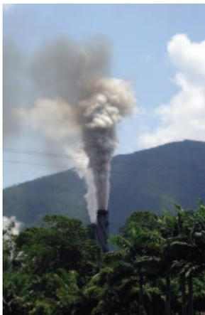
In addition to CO<sub>2</sub> and other gases, considerable amounts of particulate matter are emitted into the atmosphere by various industrial facilities, including this sugarcane processing plant in Queensland, Australia. PHOTO BY RETO GIERÉ
