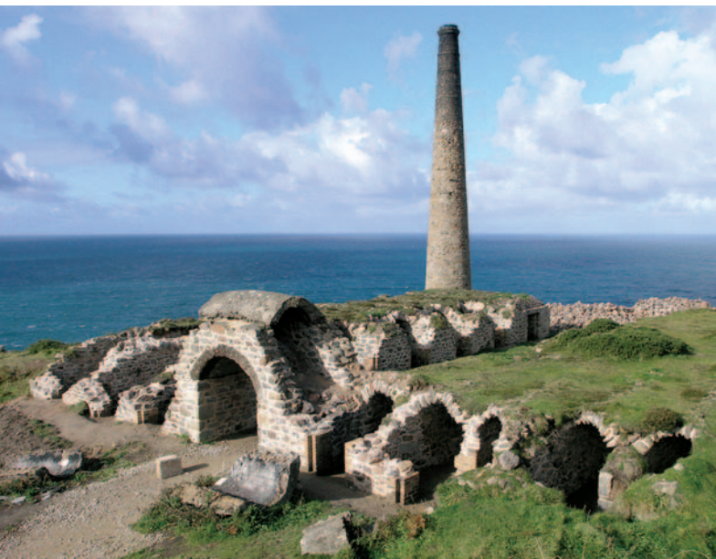
FIGURE 2 The remains of structures (lambeth flues) used to roast and drive off the arsenic from the ores mined for tin in Cornwall during the 19 th century. This archaeological heritage site is at Botallack in West Cornwall. PHOTOGRAPH COURTESY OF THE COUNTY OF CORNWALL AUTHORITIES
